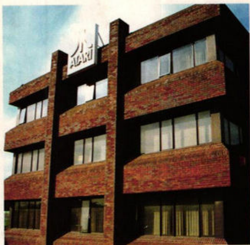
● In this building in Slough, they've found a use for those Atari power-packs. They use them as doorstops!
