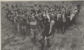
Derek Maxwell and 100 fellow diggers attack the green field site of the new headquarters
